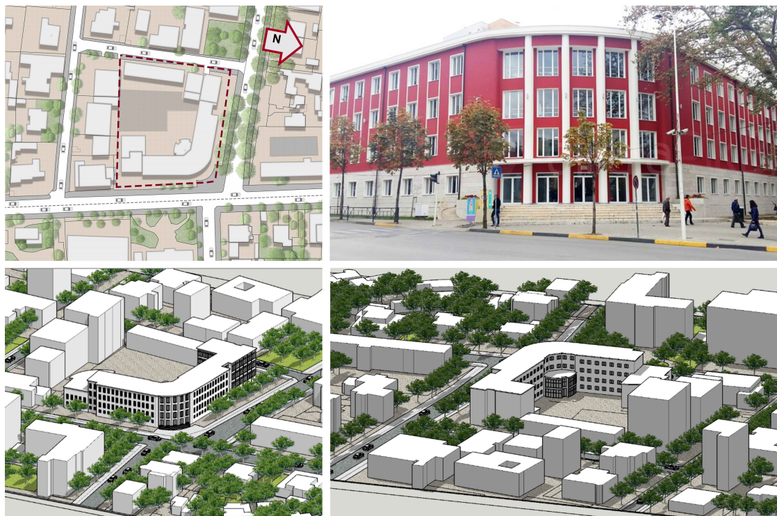
Fig. 3. Location of the 'Jordan Misja' art school (left, top), school photo (right, top) and 3D model of the school within the urban environment (bottom).
