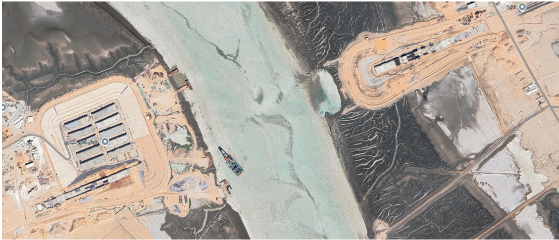
Fig. 2. Aerial view of the Khor Al Zubair Immersed Tunnel showing the surrounding geographical context and the locations of the Al-Faw and Umm Qasr portals.
