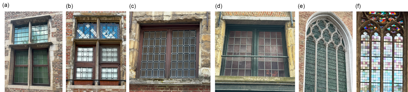
(a) Green-tinted glass with square leaded panes, Belgium, Antwerp (b) Clear glass with diamond-shaped leaded panes (top) and square lattice leaded panes (bottom), Belgium, Antwerp (c) Clear glass (with a slight smoky hue) with rectangular lattice leaded panes, Belgium, Antwerp (d) Reddish-tinted glass with square leaded panes, Belgium, Antwerp (e) Green-tinted Gothic-style stained glass with diamond-shaped leaded panes, Belgium, Brugge (f) Multi-colored Gothic-style stained glass with square leaded panes in the lancets and irregular tracery panels, Austria, Vienna
