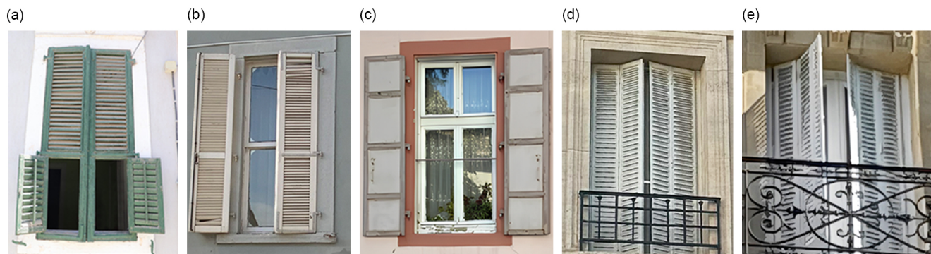
(a) Two-panel wooden slatted shading element with independently operable upper and lower sections, Turkey, Izmir (b) Two-panel wooden slatted shading element, Turkey, Izmir (c) Two-panel metal shading element, Turkey, Izmir (d) Four-panel full-height metal slatted shading element for balcony window, France, Paris (e) Six-panel full-height metal slatted shading element for balcony window, France, Paris
